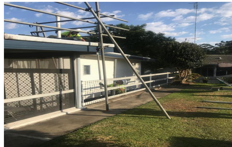
Figure 4 – Example of erected roof rail / support brace
