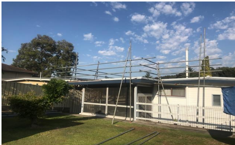
Figure 3 – Example of erected roof rail.
