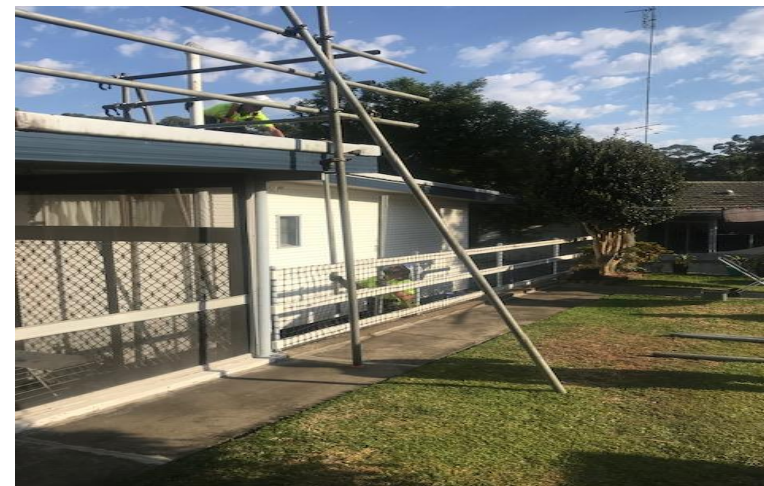
Figure 4 – Example of erected roof rail / support brace
