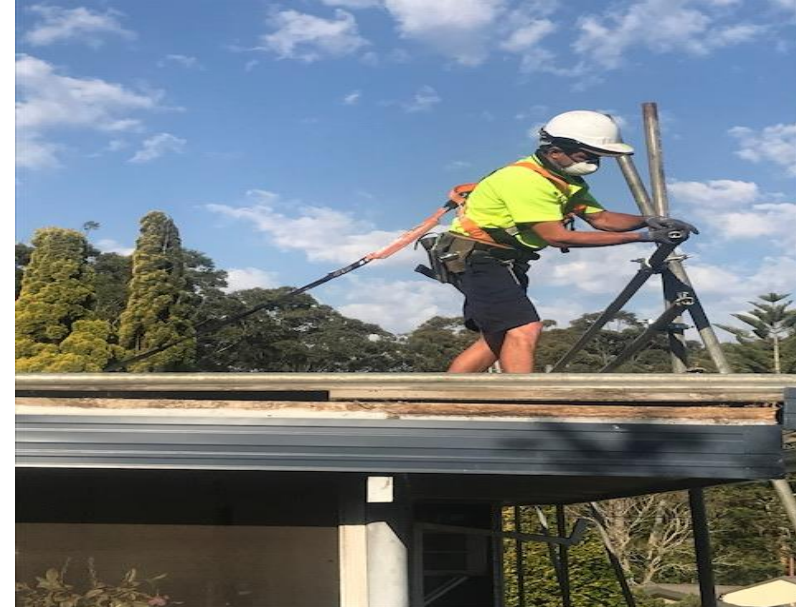
Figure 2 – Example of correct PPE / fixing coupler.
