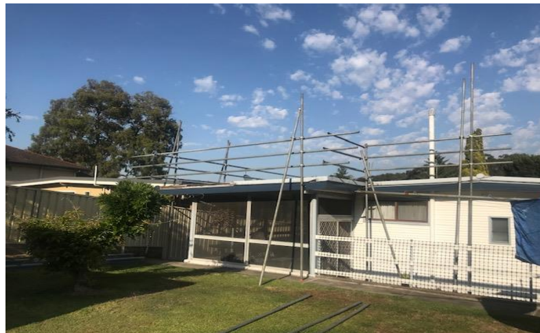
Figure 3 – Example of erected roof rail.
